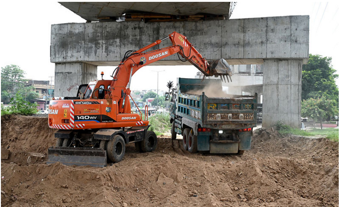
Heavy machinery is being used for the construction of a flyover along the under-construction 10th Avenue as part of ongoing development work in the Federal Capital
